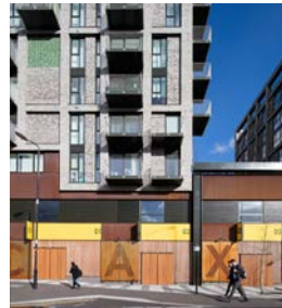
Workshops and businesses at street
