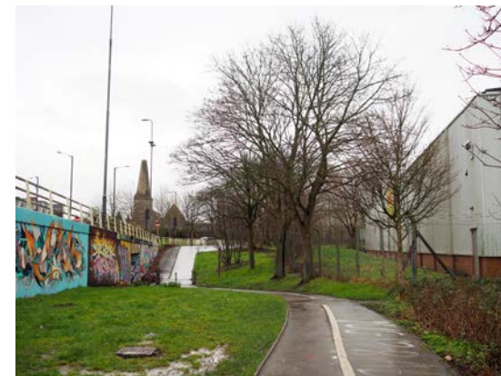
Universal House & Easton Way underpass
