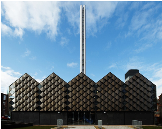
Heating Infrastructure Energy Centre, University of Liverpool
