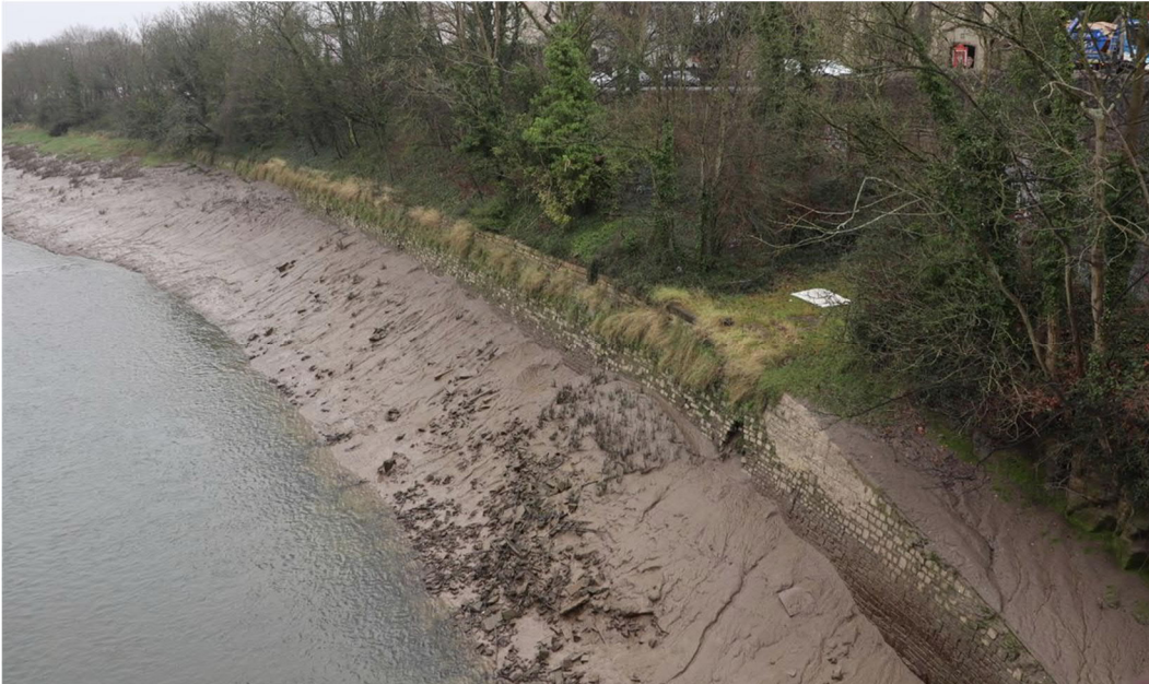
Figure 12.3: NCS18 View from Gaol Ferry Bridge looking upstream
