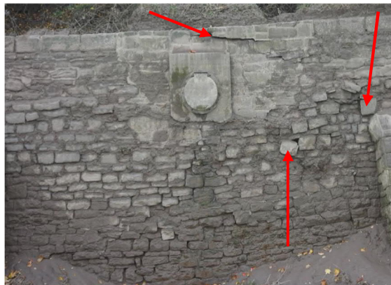
Figure 10.20: NCS28 Outfall area 2022
